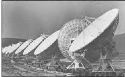
Figure.1.2 Steerable parabolic dish antennas
